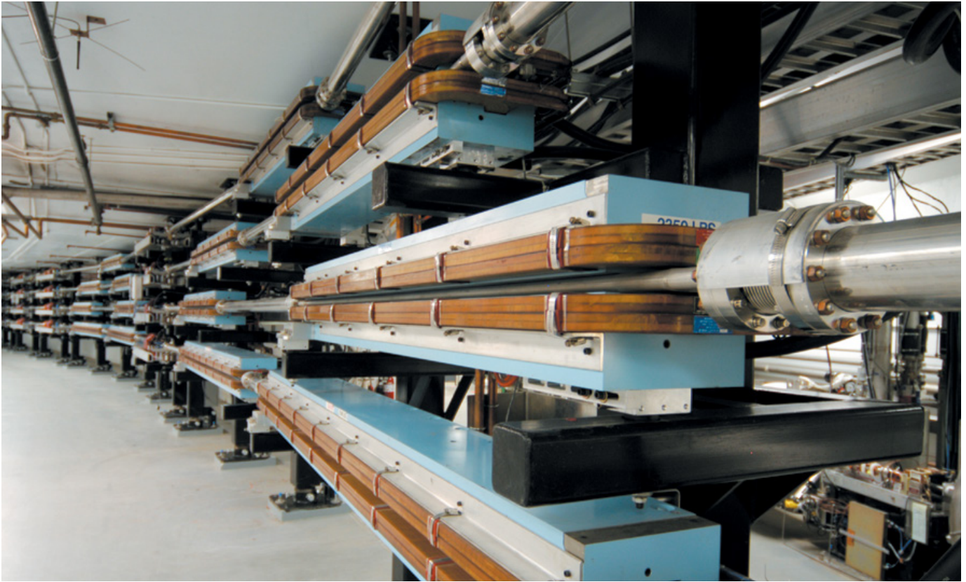
Magnets direct particles through the Continuous Electron Beam Accelerator Facility (CEBAF) at the Thomas Jefferson National Accelerator Facility.
