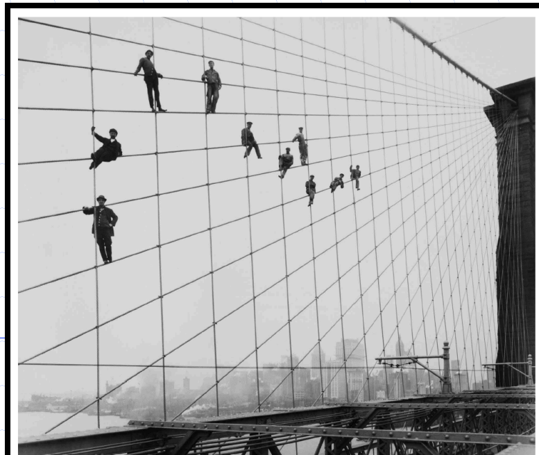
Brooklyn Bridge showing painters on suspenders. By Eugene de Salgnac, October 7, 1914. From NYC Municipal Archives. Public domain image.
