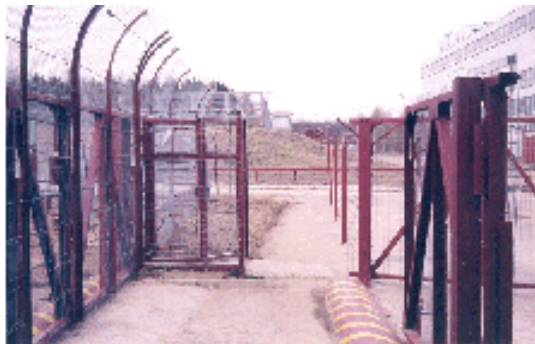
Example of enhanced security systems at Russian Ministry of Defense nuclear storage sites that are provided by the US.
