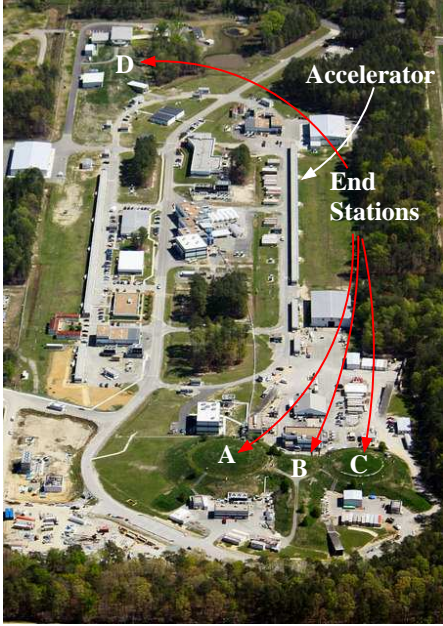
Fig 2. Jefferson Lab site.
