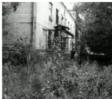
Building at the Kurchatov Institute housing HEU with no motion sensors, detectors, or portal monitors.
