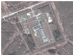
Fissile Material Storage Facility at Mayak financed by the US Cooperative Threat Reduction program.
