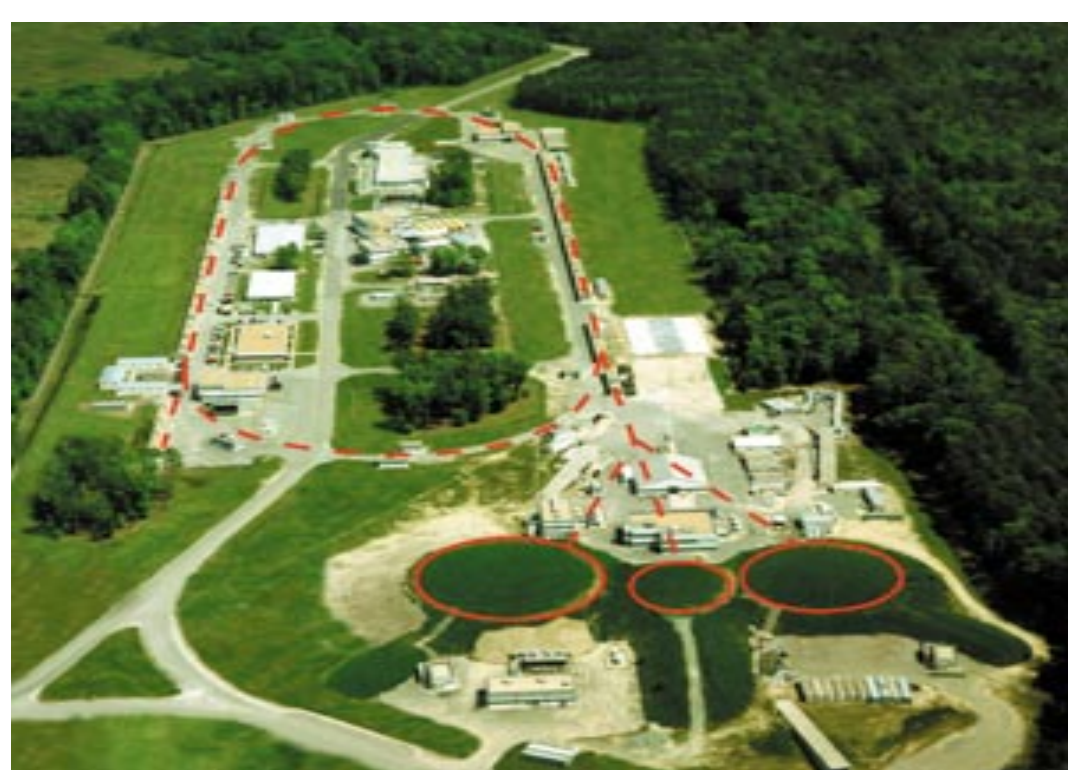
Figure 1: Jefferson Laboratory in Newport News, Virginia
